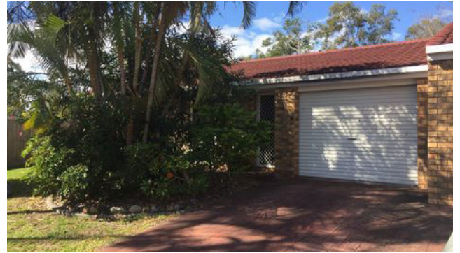
6/24-32 Old Pacific Highway UNIT $485,000 2 Bed 1 Bath 1 2024-02-12
