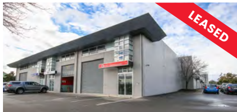
Bowden 23 Drayton Street Build area: 304 sqm
