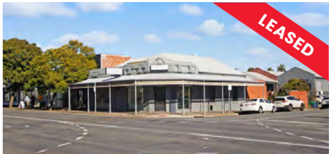
Unley 76 Unley Road Build area: 180 sqm
