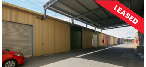
Kilburn Shed 1, 14/555 Churchill Road
